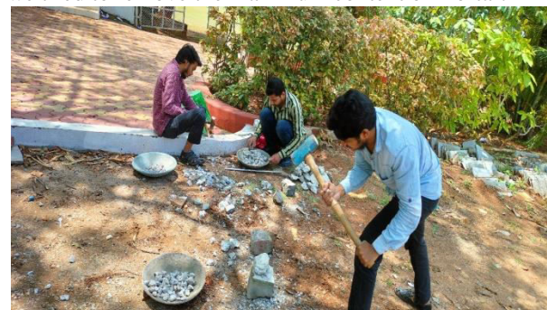
Fig 3 : Separation of coarse aggregate from demolished concrete
