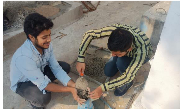
Fig 6 : Filling of concrete
