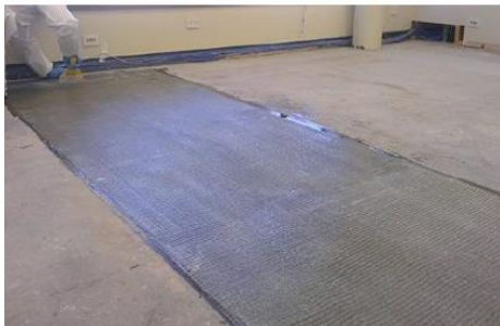
Figure No. 4 FRP Composite Strengthening services Concrete solutions
