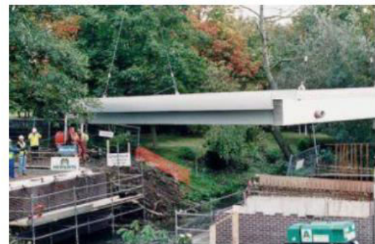
Figure 3.2 Installation of West Mill Bridge
