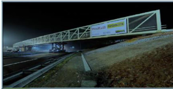
Figure 3.3 A27 Lunette FRP hybrid bridge
