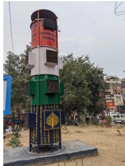
Figure 3: Smog Tower installed in Delhi
