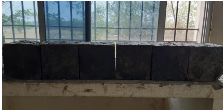
Fig. 4: Concrete mould after demoulding.
