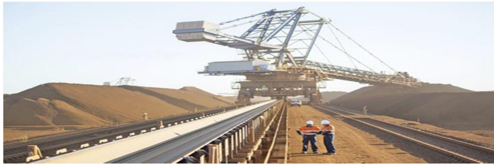
Fig.1 The belt conveyorsystem(3)
