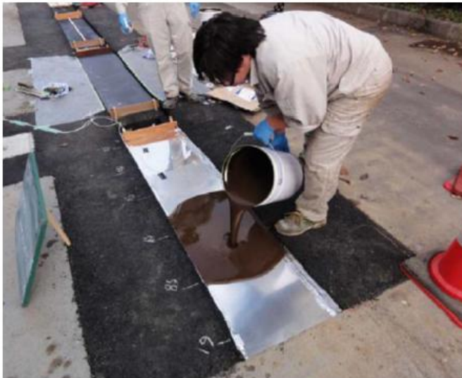
Fig-7: Photograph showing the paving of the test road
