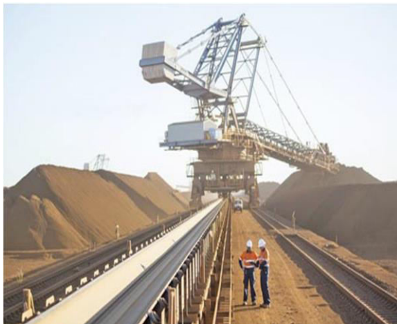
Fig.1 The belt conveyor system
