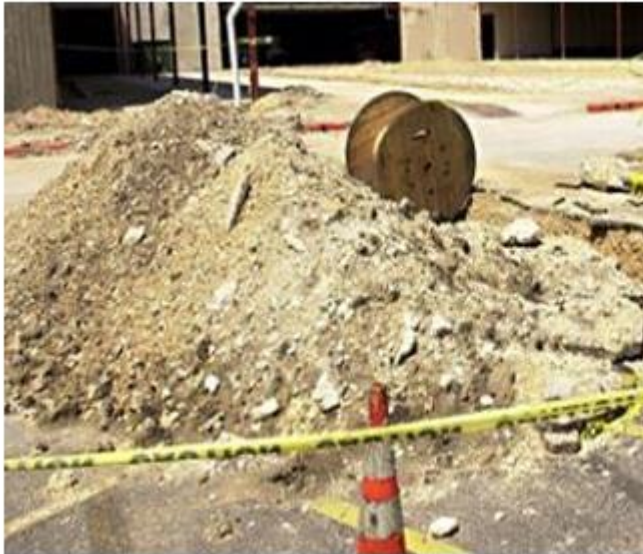
Fig.3.1. Recycling of Concrete from C&D Wastes.
