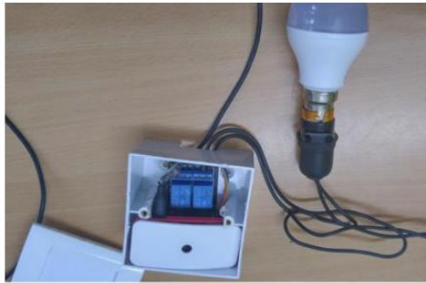
Figure 9- The picture above shows the physical connection enclosed into a box
